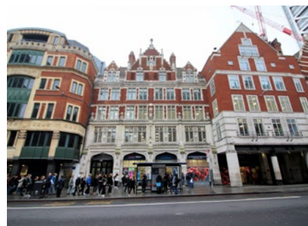
Examples of buildings within this typology Fig. 54 162 Bishopsgate Grade II | Late C19
