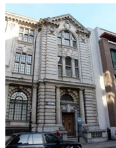
Fig. 36 King Edwards Buildings Post Office Grade II* | Early C20
