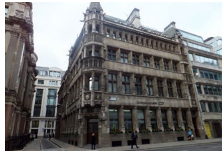
Fig. 50 13 & 15 Moorgate Grade II* | Late C19
