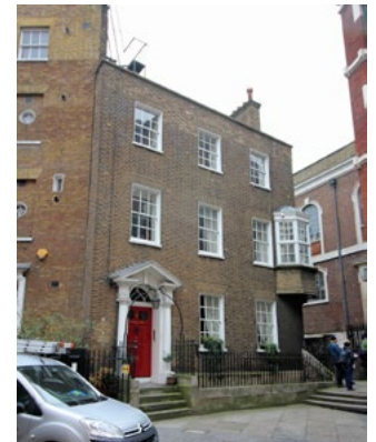
Fig. 45 The Rectory Grade II | Late C18
