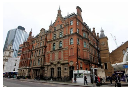
Fig. 52 Former Great Eastern Hotel Grade II* | Late C19
