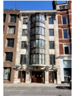
Fig. 34 Snowhill Police Station Grade II | Early C20
